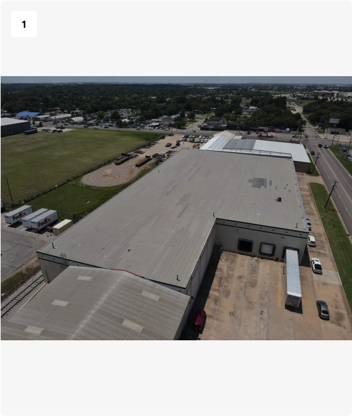
Overview of roof inspected
